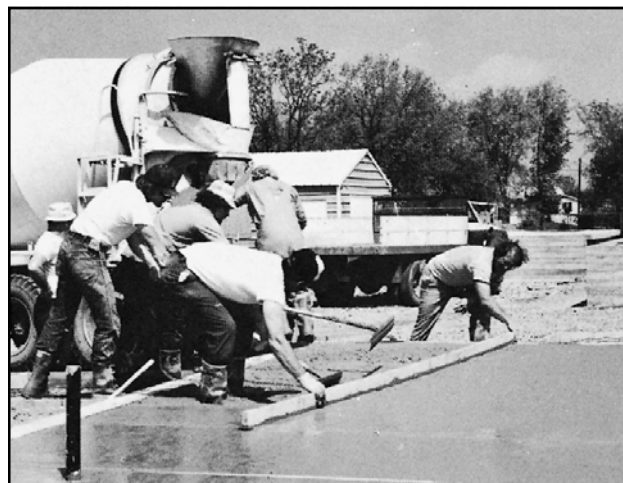
Finishing Concrete Flatwork
