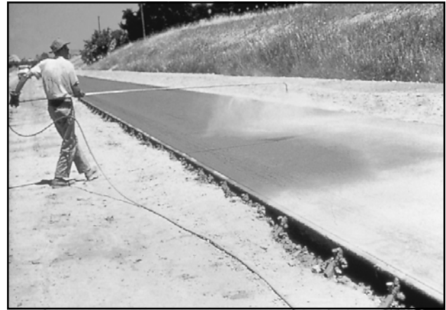
Application of liquid membrane-forming compound with hand sprayer.
