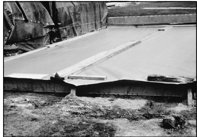
Slab on grade covered with waterproof paper for curing.
