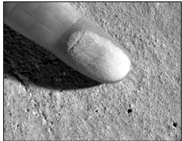
Dusting concrete surface
